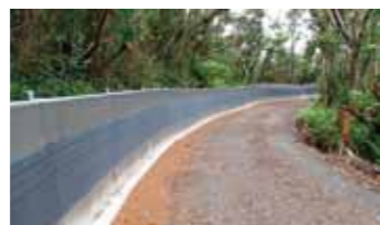
マングース北上防止柵 Fence to prevent mongoose from migrating north
